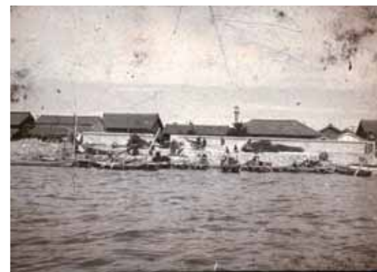
かつての前芝集落の堤防 Former bank in front of the Toyogawa floodway
