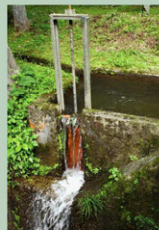
用水 (取水口) Irrigation canal (intake)
